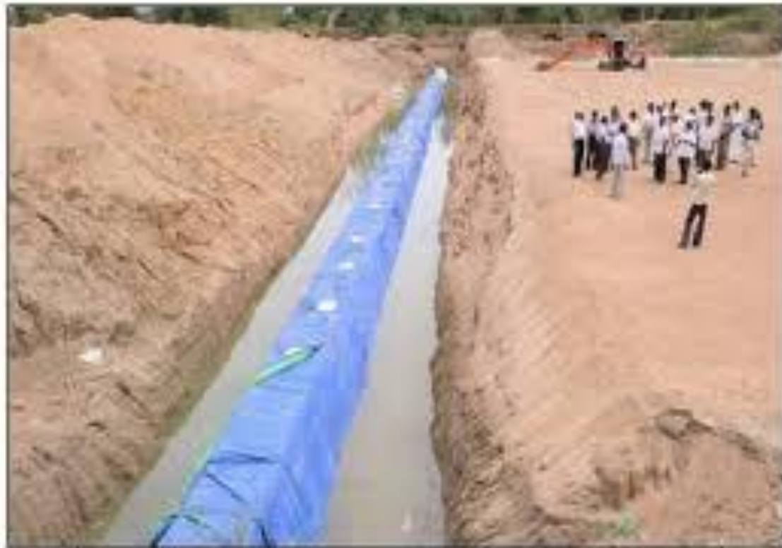
SUB-SURFACE DYKE BEFORE BACKFILLING
